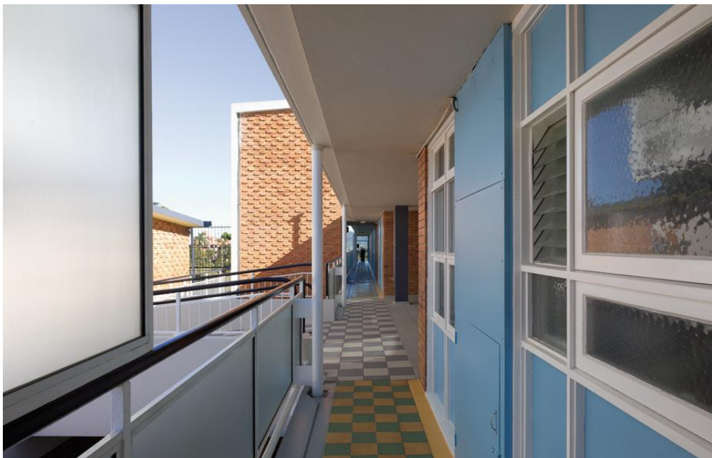
Access balconies at Torbreck
