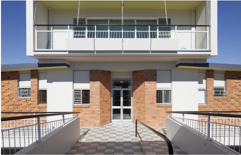
Chequerboard paving in different colours identifies each level
